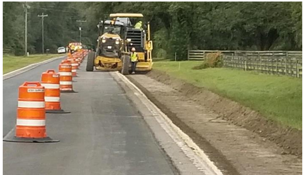
C 478 Widening from US 301 to SR 471
