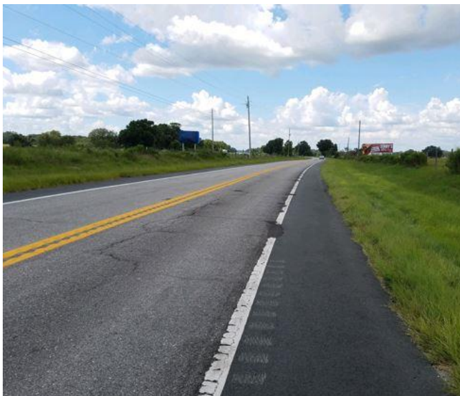
[After Shoulder Widening]
